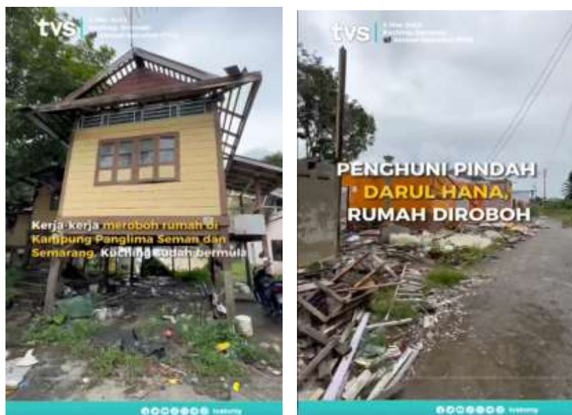
Figure 1. Demolition of houses in Kampong Seberang on the north bank of Sarawak River, opposite Kuching Waterfront, as reported in March 2023. (Source: Ahmad Nasrullah, 2023).
