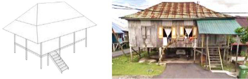
Figure 7. The hipped roof form of potong limas type is said to emerge during the Brooke period. Source: Author's fieldwork.
