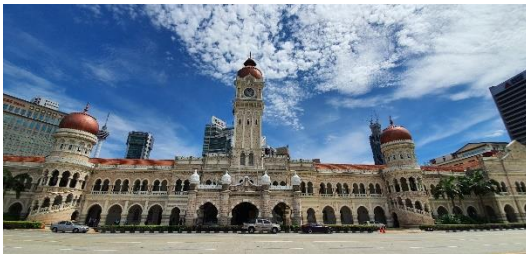
Figure 2: Sultan Abdul Samad Building (Source: Authors)
